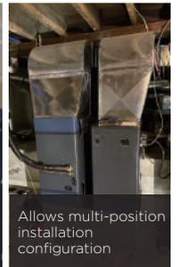
Allows multi-position installation configuration
